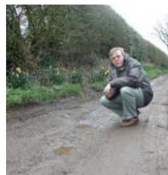
Barry Stamp inspecting the poor state of Back Lane
