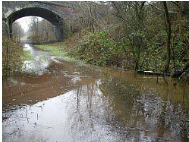
Excess water from the old railway line is flooding Station Road, Haughton
